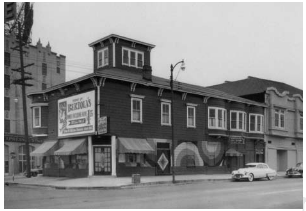
Bertola's Restaurant (demolished), Pezzola's Block, Telegraph and 46th St., 1953.
